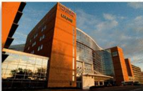
University Hospital Little Rock, Arkansas
