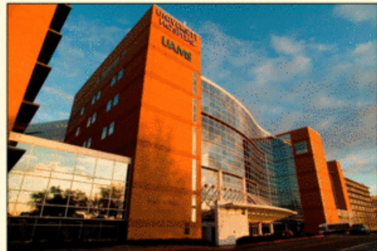
University Hospital Little Rock, Arkansas
