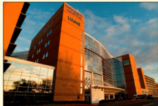
University Hospital Little Rock, Arkansas
