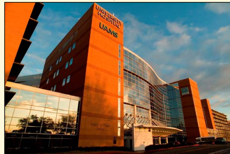
University Hospital Little Rock, Arkansas
